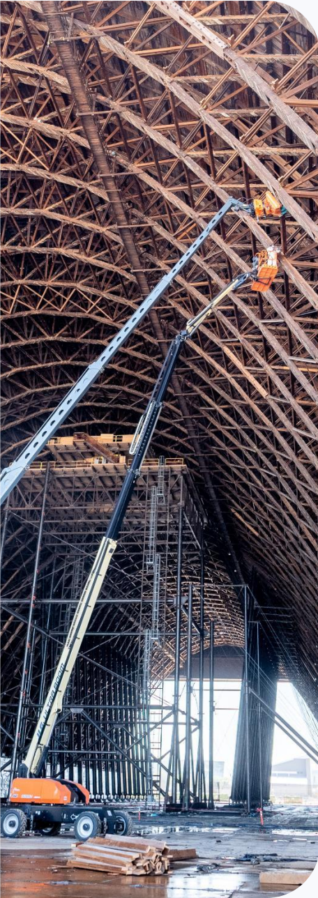
Temporary steel pillars supporting the Hangar 3 structure.
