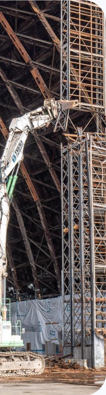
Multiple pieces of heavy machinery, including a high-reach excavator, collaborate to tear down the massive wooden sections of the hangar.
