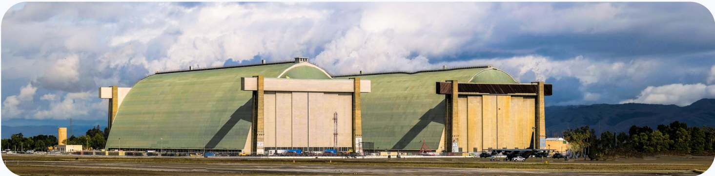
Exterior view of Hangars 2 & 3 at Moffett Field.
