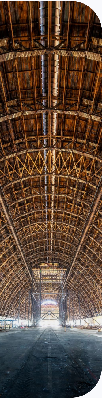
The intricate wooden framework of the hangar stretching down its entire length.
