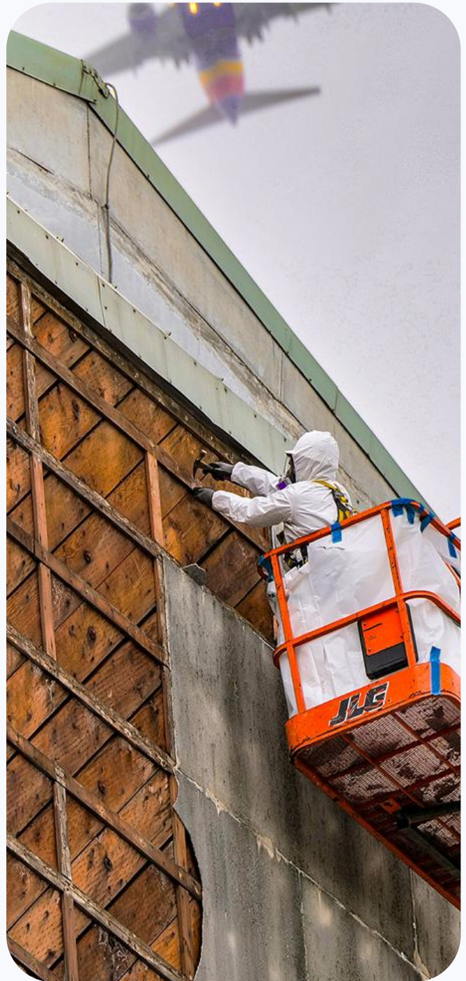
A worker in protective gear removes the exterior cladding above a hangar door.
